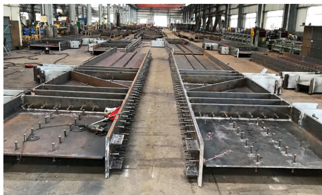
鋼板梁製造 Steel Plate Girder Fabrication
